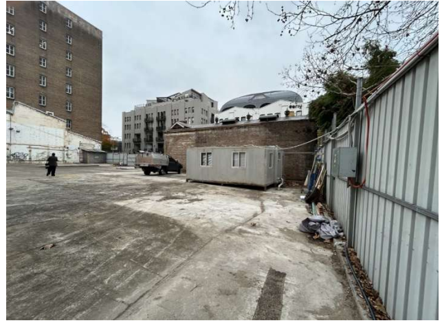
Figure 12 - View northwest showing in ground drainage connections and hardstand concrete.
