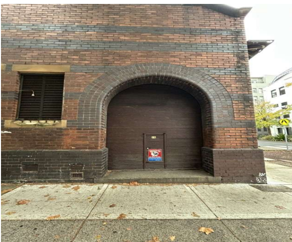
Figure 9 - The electricity Substation roller door entrance with masonry detail archway.
