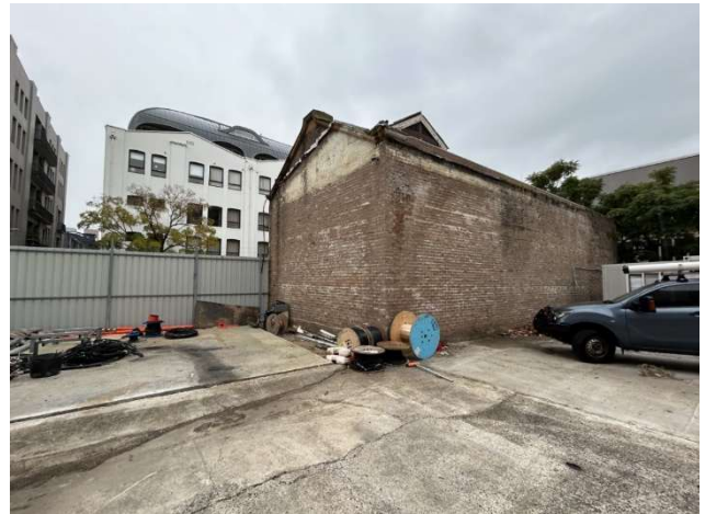
Figure 14 - Detail of the rear façade of the electricity Substation, facing northeast.
