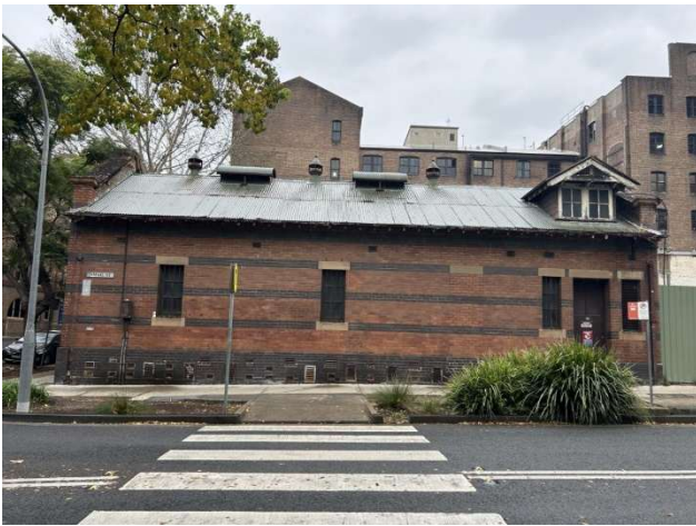
Figure 5 - View south showing the northern elevation of the electricity Substation.
